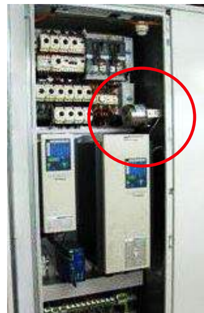
Individual cabinets protected to focus on specific hazards
