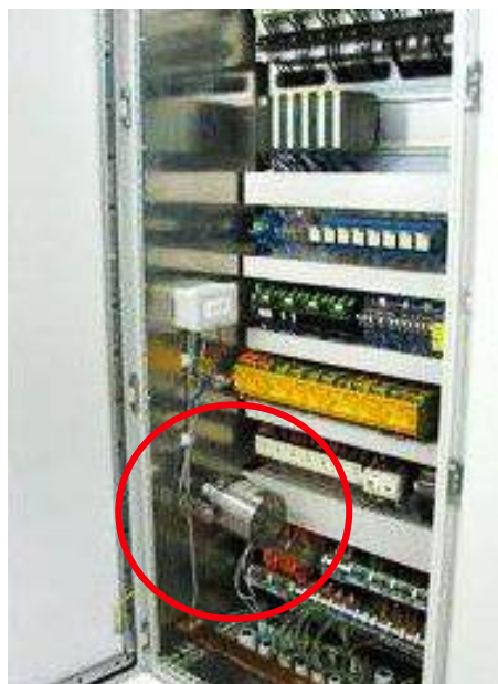
Individual cabinets protected to focus on specific hazards
